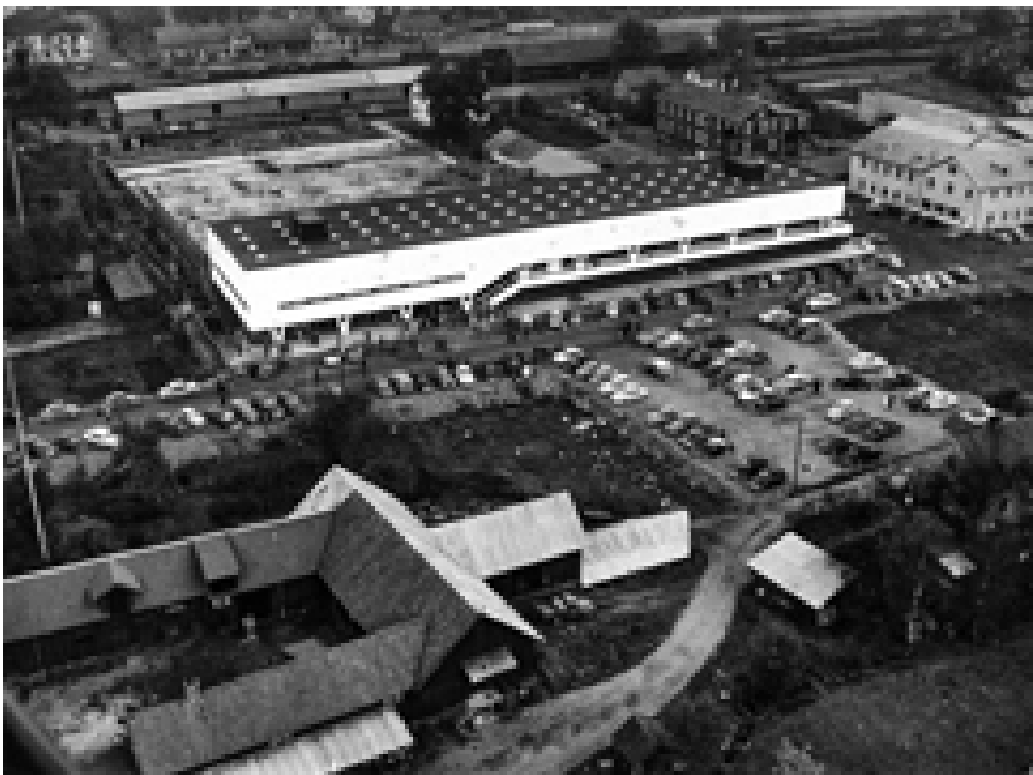
Terrain in Älmhult, 1959. The grey building in the upper right corner is the Lagerblads Snickerifabriken. The modernist white building is the 1958 store and we can see the construction of the 1960 extension behind it. The building was designed by architect Claes Knutson and today it is used for the IKEA Museum (© Inter IKEA Systems B.V.)
